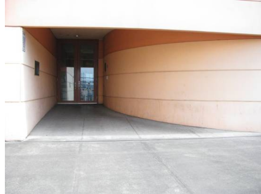
Rear entrance located on north side of building (356A).
