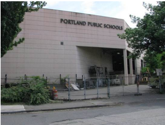
North elevation of building (356A).
