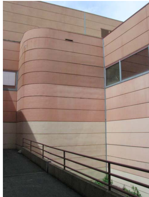
Rounded edge to building located near main entrance (356A).
