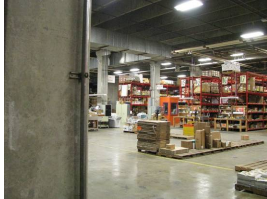
Interior of warehouse section of building (356A).
